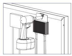
3) Tighten the mounting bolt on the MLPE Frame Attachment Kit to 12 lb-ft (144 lb-in).
